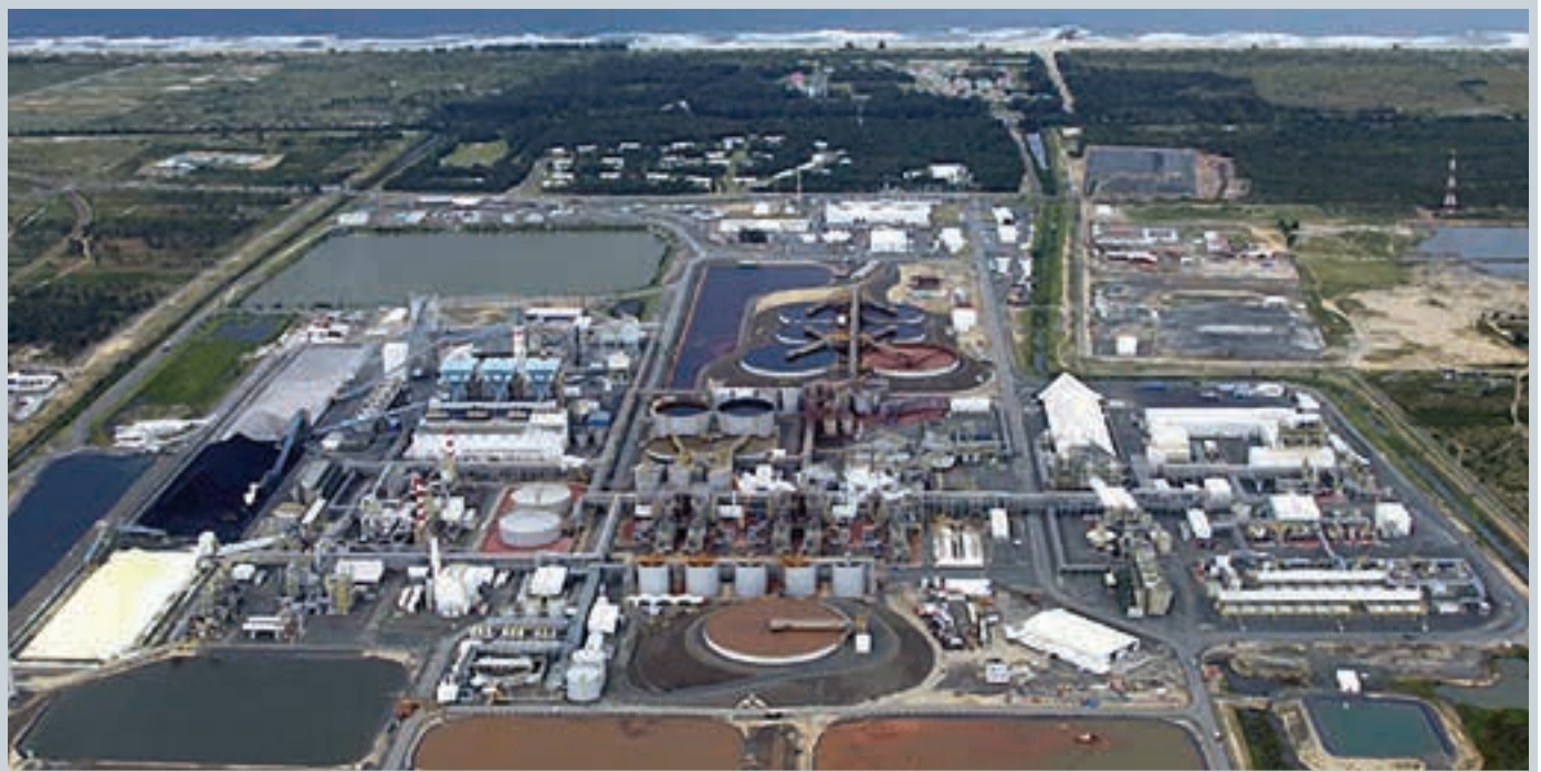
Aerial view of the Ambatovy nickel-cobalt HPAL and refinery, in Madagascar
